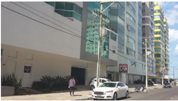
Figure 4 12-story tall buildings with base glued to the side boundaries and overlapping towers with side setbacks
