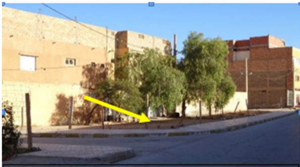
Figure 2 part of public space fenced and added to the house.
