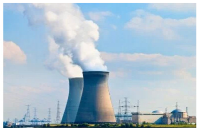
Figure 6 Water vapor from the cooling towers of nuclear power plants.
