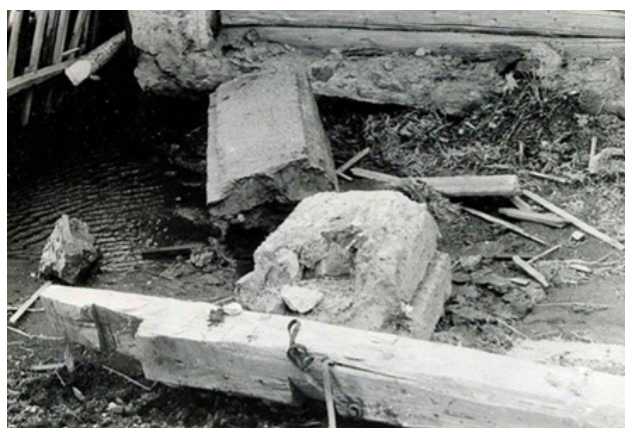
Figure 3 Concrete pillar torn by ball lightning. 18
