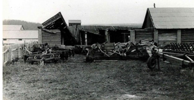
Figure 2 A barn destroyed by ball lightning. 18
