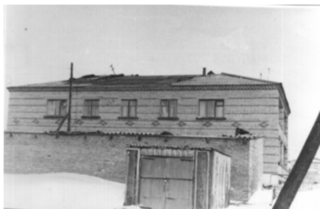
Figure 1 The roof of a two-story house destroyed by ball lightning. 17
