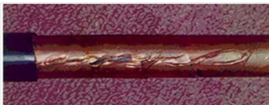
Figure 7 Damaged or Cracked Copper Screen.
