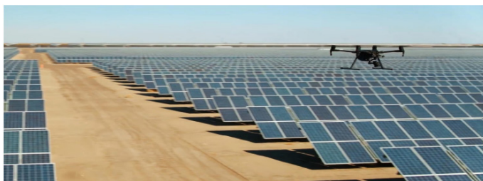
Figure 24 A RaptorMaps Drone Inspecting a PV Power Plant. Reprinted from Raptor Maps. 84
