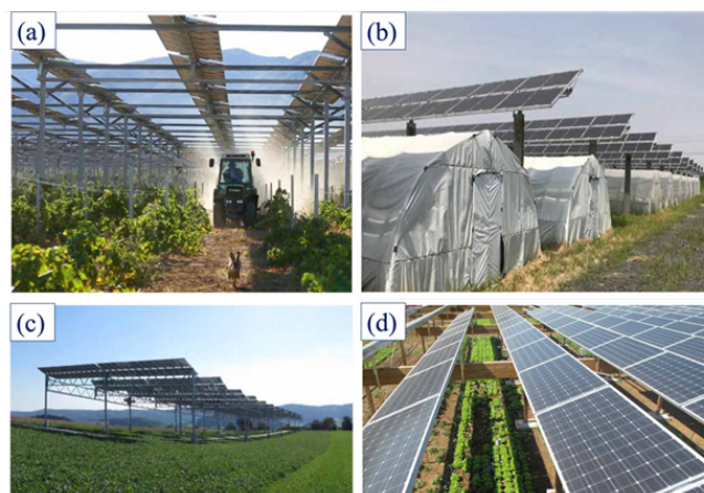
Figure 16 The demonstration of (a) Elevated agri-photovoltaic plant, (b) tunnel types greenhouses agri-photovoltaic and (c) and (d) Orchard Agri-photovoltaic plant. The figure is regenerated from Ref. 71
