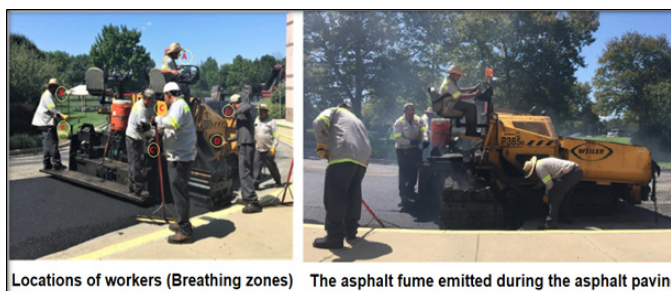
Figure 4 Workers during the asphalt paving process.
