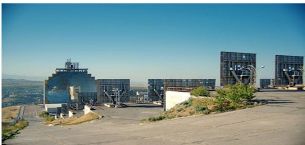
Figure 1 Big Solar Furnace with a thermal power of 1,000 kW in Uzbekistan (Parkent).
