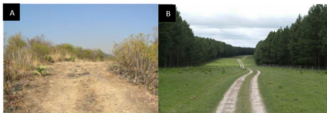
Figure 7A and 7B The construction of firebreaks is important in any afforestation and reforestation project.
