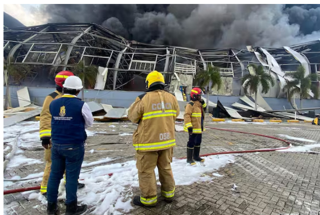
Figure 7 Fire at Cartagena container terminal.
