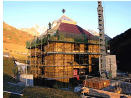
Figure 7 Construction of a house with straw bale walls in Switzerland. 6
