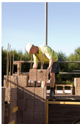
Figure 1 Wall with lightweight concrete blocks of wood chips. 1
