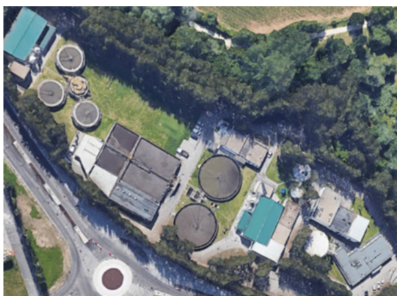
Figure 3 Aerial view of the Olhalvas WWTP.
