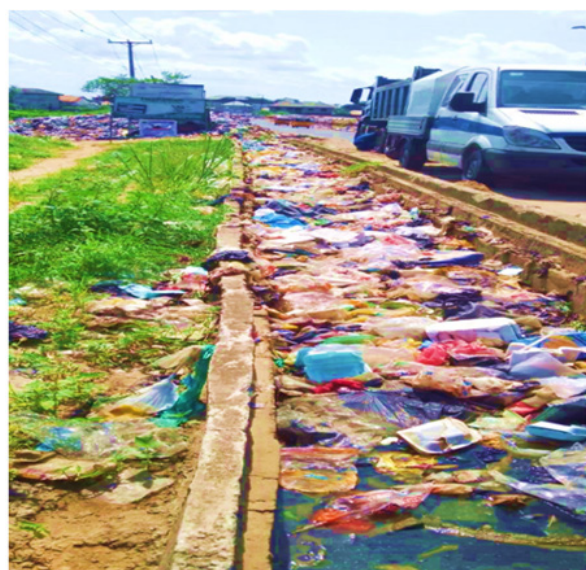
Plate 2 Solid waste dumped in drainage facility along St. Johns - Ogbogoro road of the study area.
