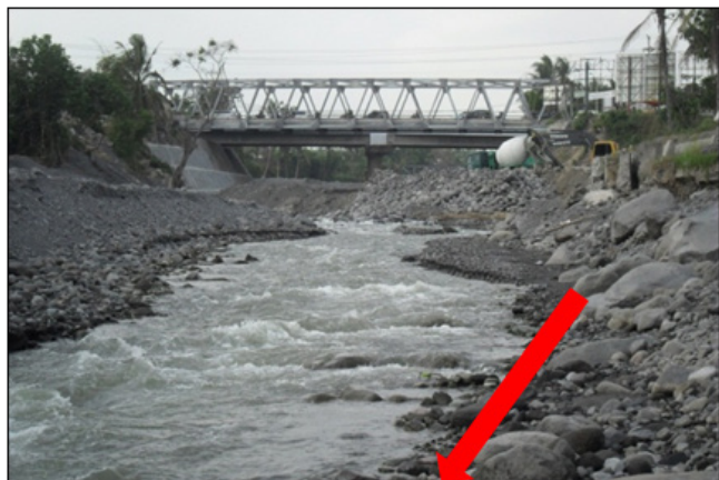
Figure 6 River condition at Pabelan Bridge.
