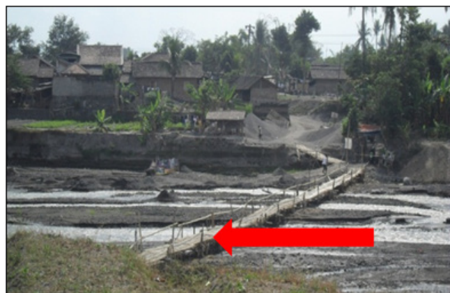
Figure 5 River condition at Srowol Bridge.
