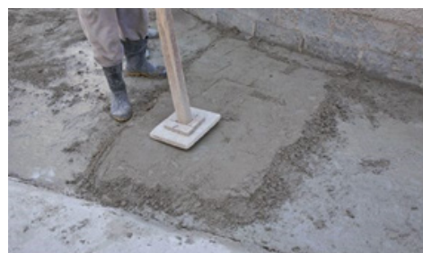
Figure 3 Exemplification of the dry and heterogeneous aspect of conventional subfloor mortar.
