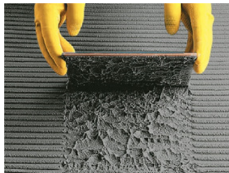
Figure 5 Exemplification of broken mortar cords promoting impregnation of the piece.
