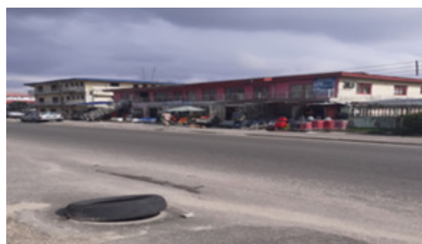
Figure 6 Residential buildings converted to commercial use at Oromenike Layout (D/Line). Source Researcher's Field Survey, 2019.
