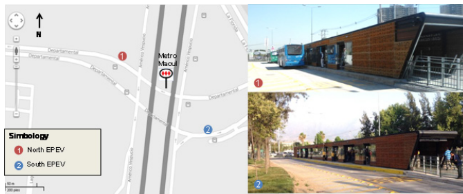
Figure 1 Characteristics and location of EPEV stations in Santiago de Chile.
