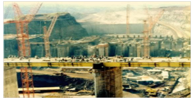
Figure 2 Photo of its construction at the time of 1980. 2
