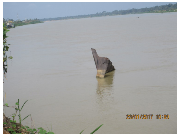
Plate 1 Collapsed sheet pile wall at Opokuma/Kolokuma.
