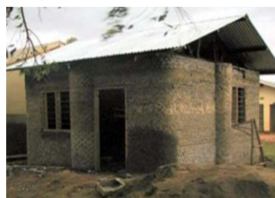
Figure 3 First bottle house construction.
