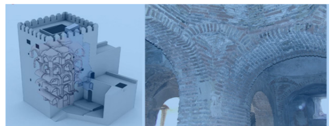
Figure 4 The systems for arches and domes in the Homage Tower. Adapted from Villegas (2012).
