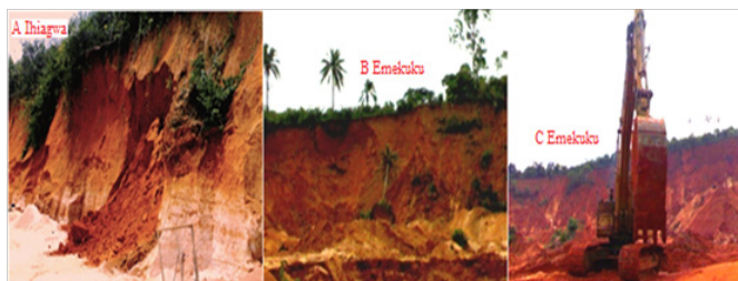
Figure 5 (A) Abandoned borrow pit showing old slide surface and recent slumping (Left). (B) Active borrow pit with rapid sliding of palm trees into the pit (Centre). (C) Heavy duty excavator at work, often affected by sliding (Right). Images created by Nwachukwu MI.
