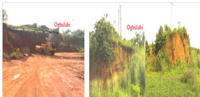
Figure 7 (A) Borrow pit operation threatens collapse of family duplex and fence (Left). (B) Borrow pit threatens high tension power pole (Right). Images created by Nwachukwu MI.
