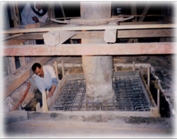
Figure 14 Soil stabilization and footing support in El-Azra church.
