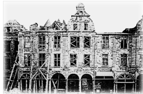
Figure 6 Main square in Paris before restoration and conservation. Courtesy of Sepedem- photographer.
