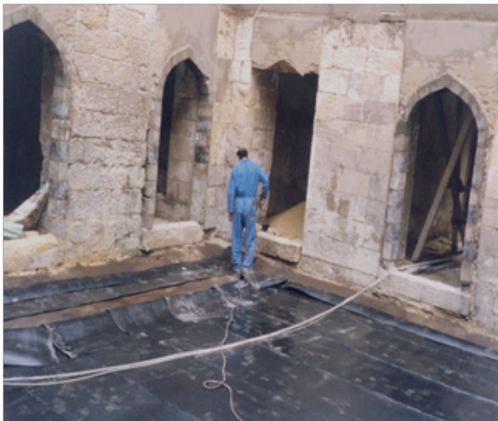
Figure 15 Floor isolation process in Sarghatmash mosque-El Saleeba Cairo.
