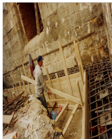
Figure 13 Soil stabilization process in El-Kekhya Mosque.
