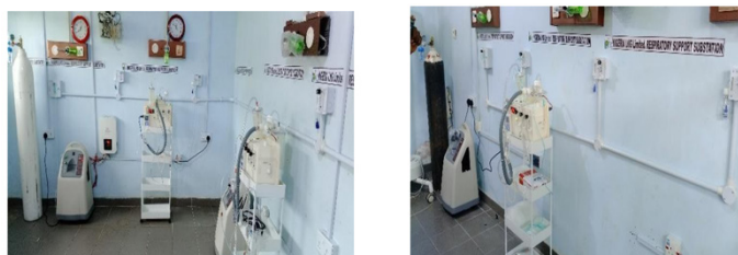
Figure 5 Two NDUTH Yenagoa Substations (left – outborn, right – inborn sections).
