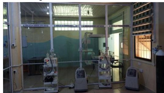
Figure 3 AKTH, Kano substation.
