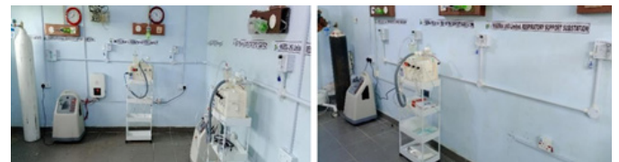
Figure 1 Two NDUTH Yenagoa Substations (left – outborn, right – inborn sections).
