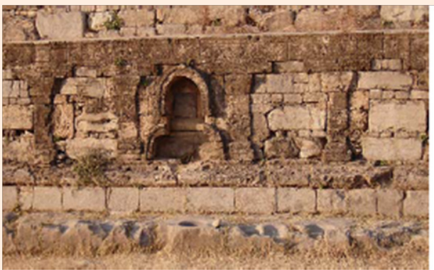
Figure 2: Wall of small stupa at Dharmarajika with thick fungal biofilm.
