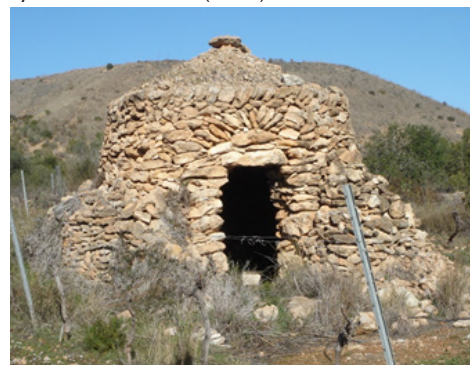
Figure 3 Dry stone hut in El Vendrell. Authors: Guillén-Villar, Abraham; Traver-Vives, Montserrat.
