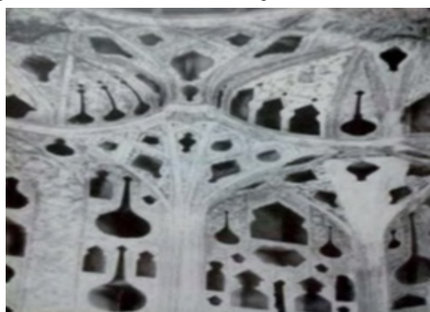
Figure 4 A view of the tongbori and muqarans work of the sixth floor wall; Source: Authors.
