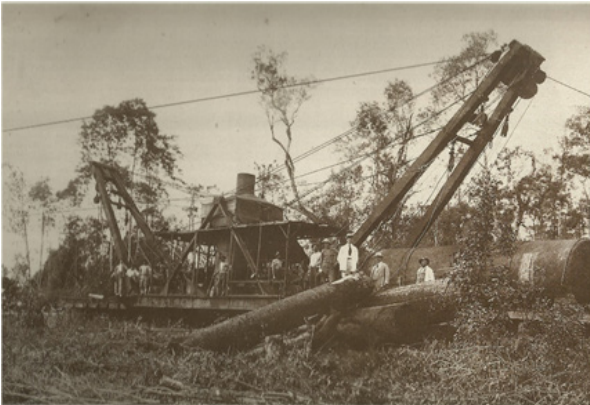
Figure 2 Cranes used to collect tree logs from the interior of the forest to the edges of the trail.
