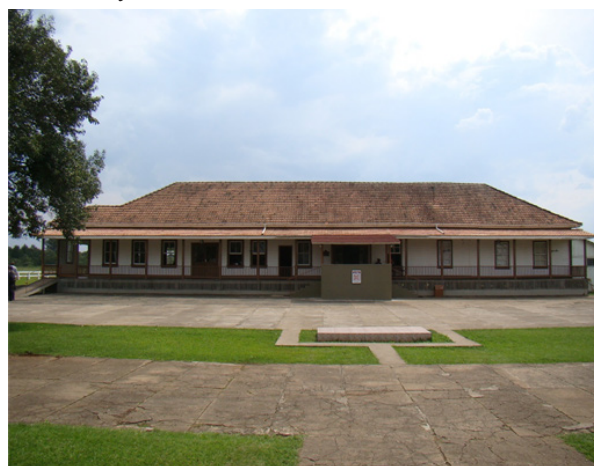
Figure 4 Management offices restored.
