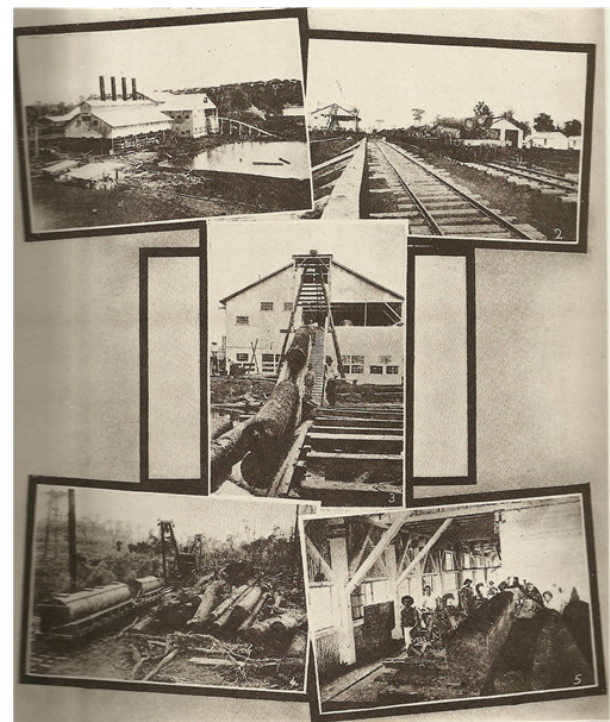
Figure 3 Scenes of the wood processing steps in the large Lumber factory in Três Barras.
