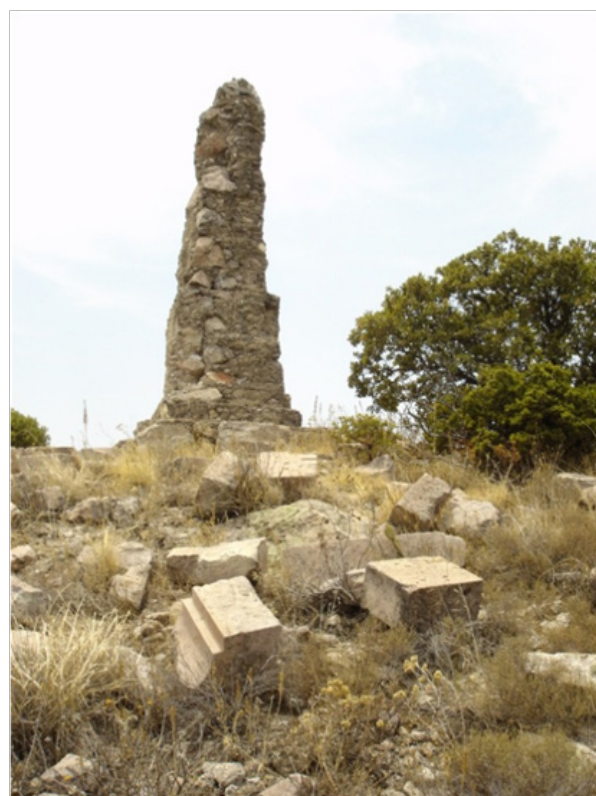
Figure 7 View of the obelisk at Fuerte del Sombrero.
