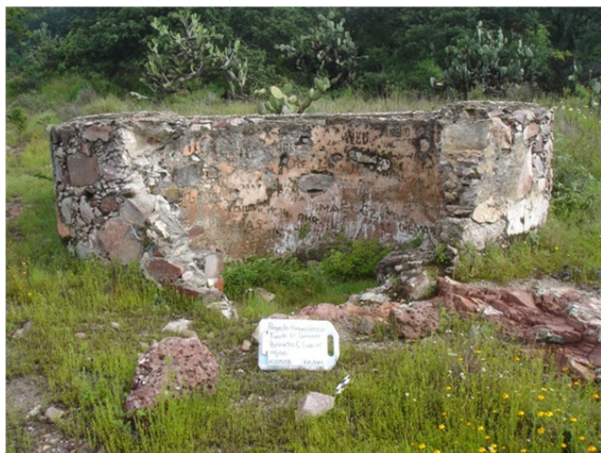
Figure 8 Cistern of stone and mortar.
