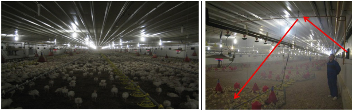
Photo 1 A flat ribbed ceiling is not a good choice for cold winter conditions (especially for small birds) due to the high speed cold draught on the bird level from the inlet, reflected from the top. At a very low outside temperature the falling air causes water condensation on the litter, triggering FPD development. At the same time this type of ceiling is very good for creating a high speed tunnel (summer) ventilation.
