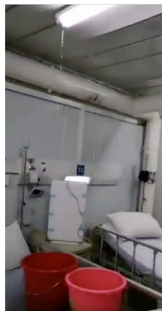
Figure 1A Example #1 still image frame from a video post of water leak.
