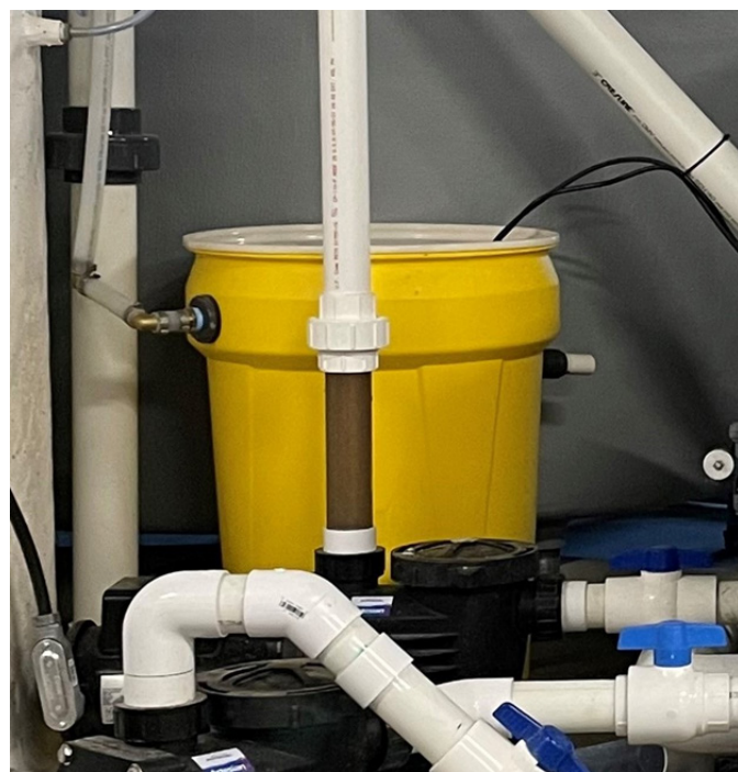
Figure 17 Sump barrel used to collect overflow from the drum filter standpipe.
