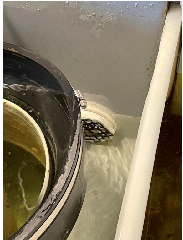
Figure 5 Combined effluents of the culture tank exiting the side drain structure.
