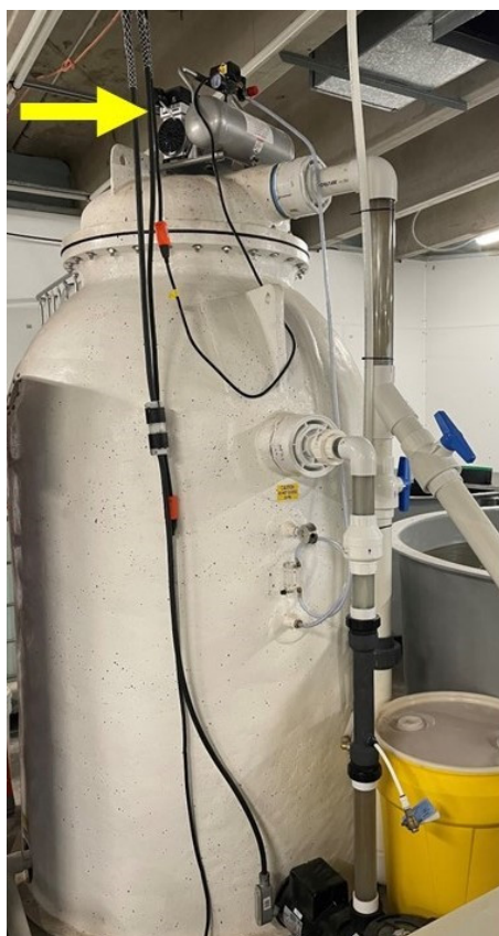
Figure 8 Air compressor on the pressurized bead filter to initiate agitation cycles.
