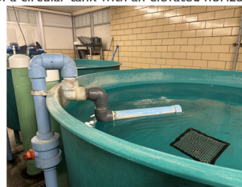
Figure 2 Image of circular tank with submerged horizontal spray bar.
