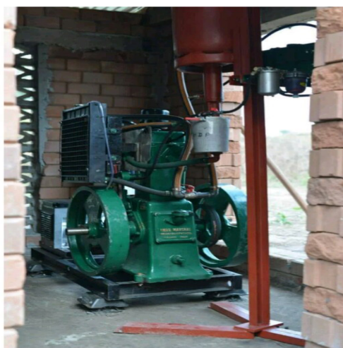
Figure 1 Image of the generator using palm oil at RMB.
