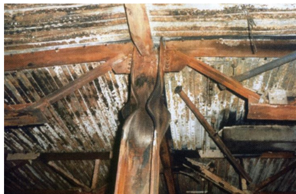
Figure 30 Example of allowable local deformation of structural support of compartment ceiling.
