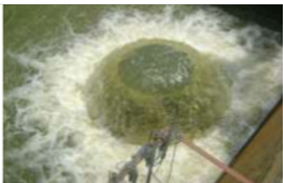
Figure 4 Balancing tank of KNWTP.
