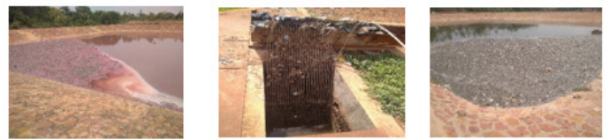
b) facultative basin c) pretreatment system: screen bar d) surface of the anaerobic basin
