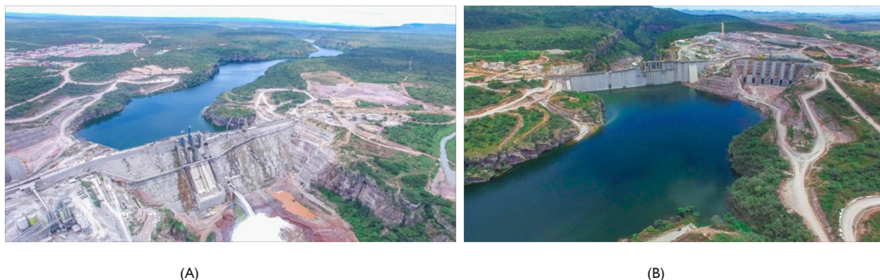
Figure 12 Reservoir filling process. (A) Downstream view of the bottom outlet operation. (B) Upstream view of the reservoir filling process. March 17 th , 2018.
