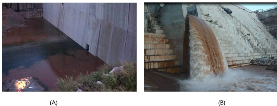
Figure 11 The first operation of the bottom outlet during the reservoir filling. A) Upstream view of the bottom outlet entrance. B) Downstream view of the bottom outlet. March 11 th , 2017.
