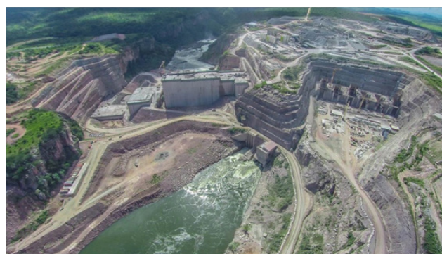
Figure 3 The second stage of the river diversion, January 21 th , 2016.
