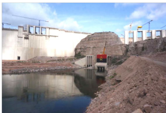
Figure 9 Upstream view of the diversion tunnels 1 and 2 after the closure of the tunnel 2. March 11th, 2017 (Source: Intertechn Consultores Associados S.A., 2017).
