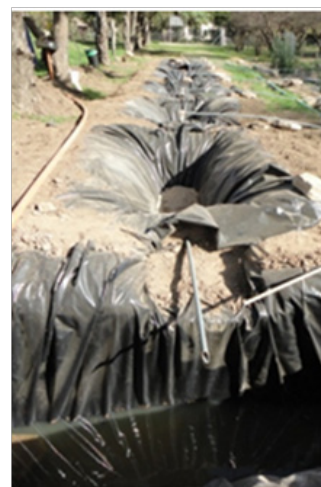
Figure 3 Construction of wetlands.
