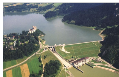
Figure 5 Czorsztyn-Niedzica dam on the Dunajec River (downstream view). 4
