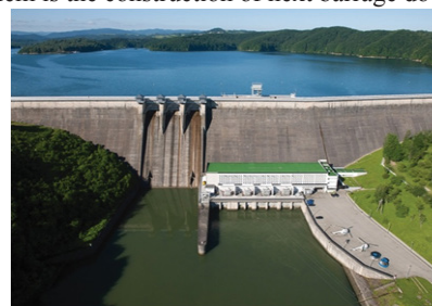
Figure 6 Solina dam on the San River (downstream view). 4
