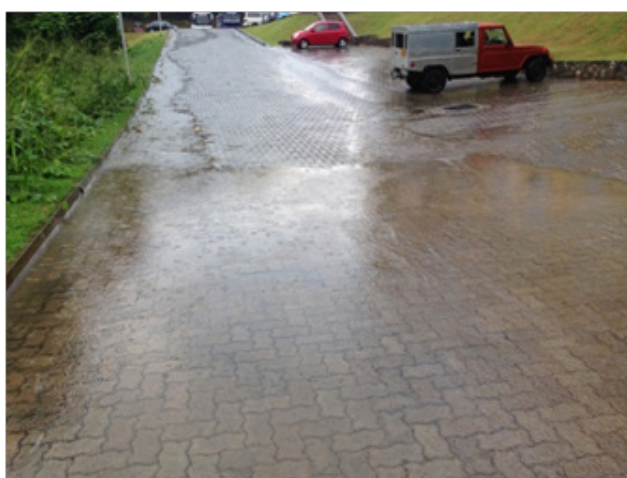
Figure 1 Water pooling in front of Faculty of Engineering due to a small rainfall. 2
