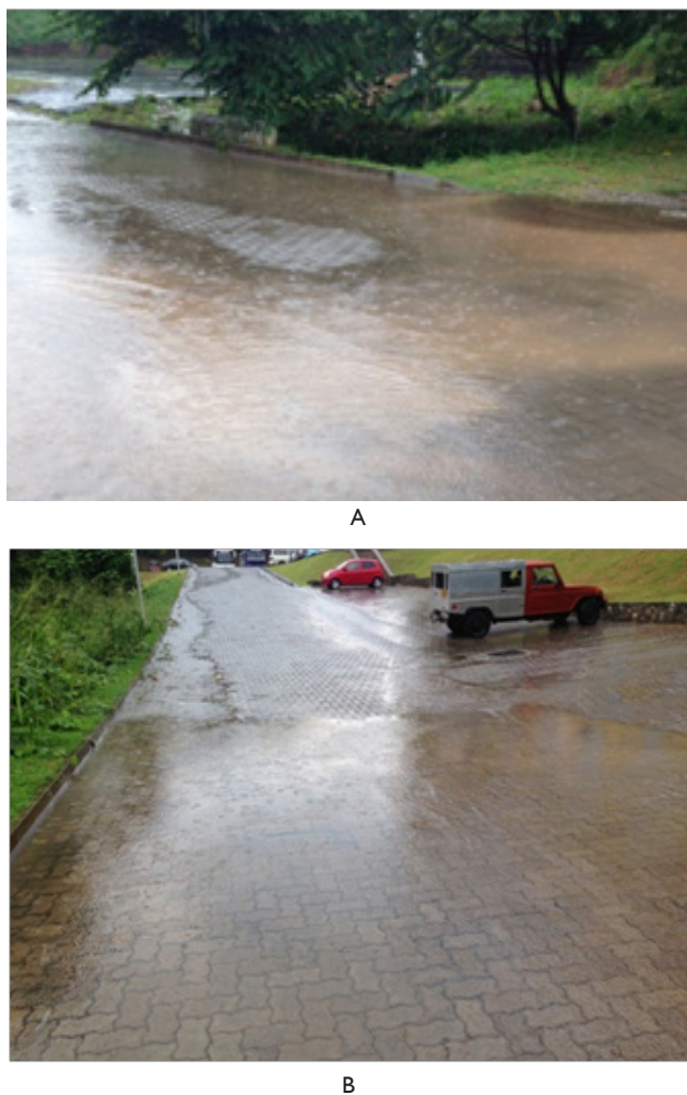
Figure 1 Water pooling in front of Faculty of Engineering due to a small rainfall. 2
