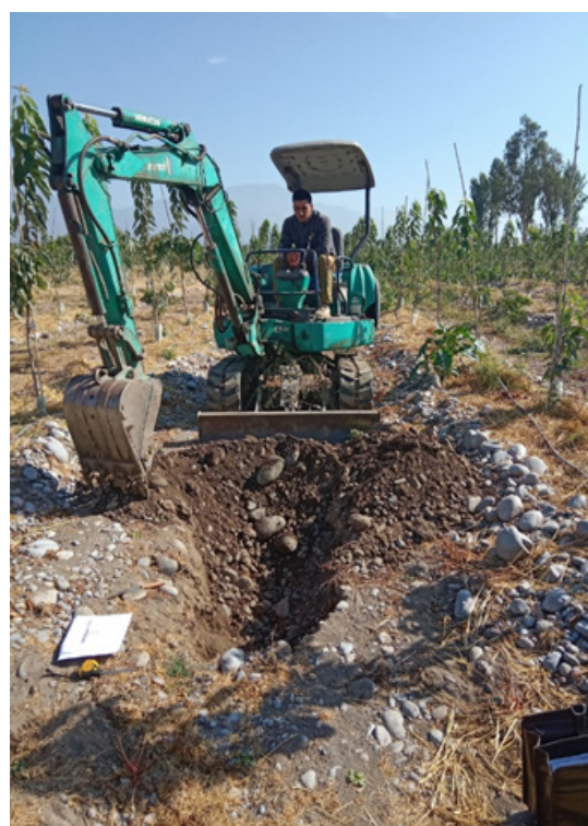
Figure 2 Excavations for soil profile description with a backhoe.
