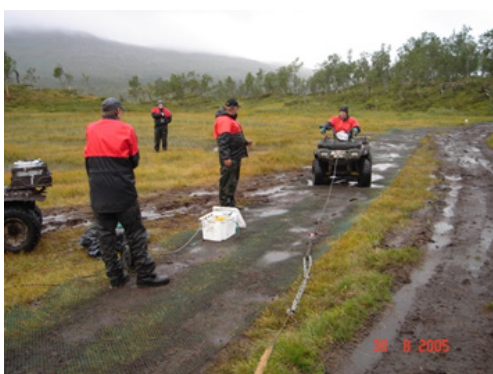
Figure 3 Pulling tests on a PP geonet side by side to the rutted old trail (to the right). The route has been passed by about 60 ATVs during work on a power dam up streams.
