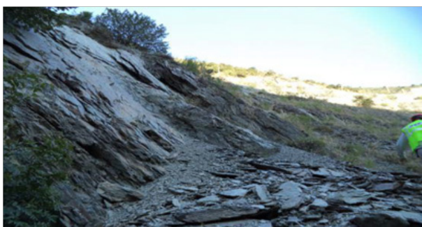
Figure 5 Dip slope about 30-40m upstream of EA-08 portal
