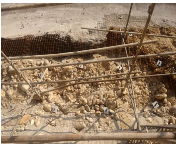
Figure 12 View of RBM & Talus/Filled Muck in TRT Outfall Area
