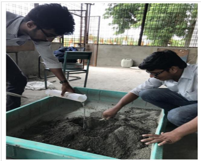
**Figure 3** Preparation of grouting mixture using hand mixing method.
