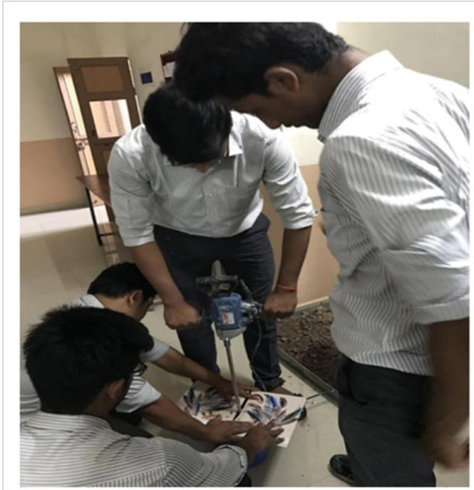
**Figure 2** Preparation of grouting mixture using mixer.
