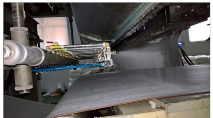
Figure 1 A water quenching system.
